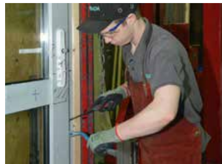
Manual glazing removal.
