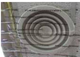
d) Sealing all ventilation is a requirement for accurate testing.
