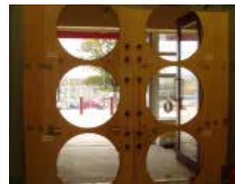
c) Installation of template to hold the fans.
